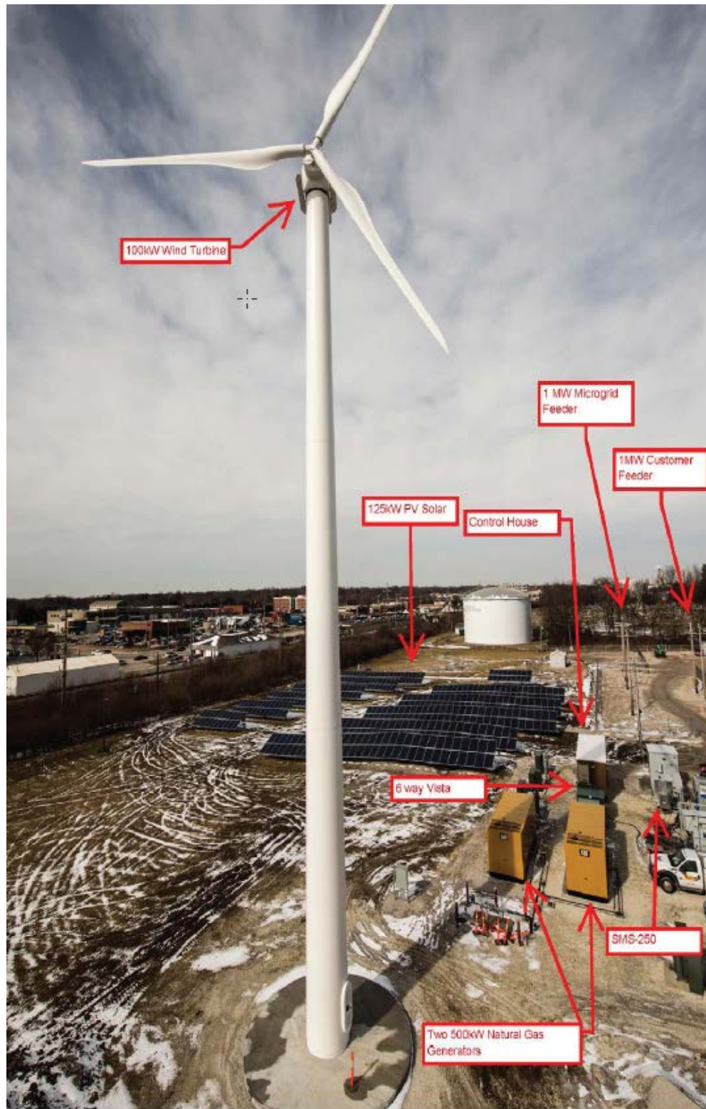
Figure 17: Ameren Microgrid Featuring Wind, Solar, Natural Gas Generator, and Battery
