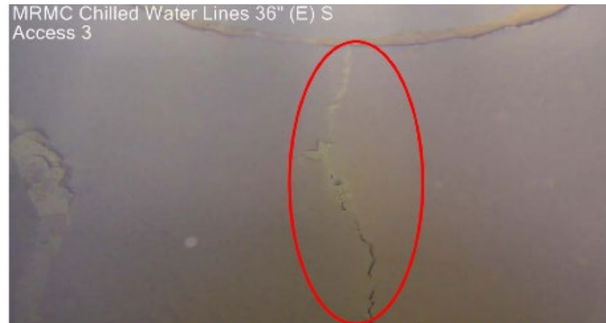
Longitudinal Crack observed at the invert of Pipe 8019 pipe
