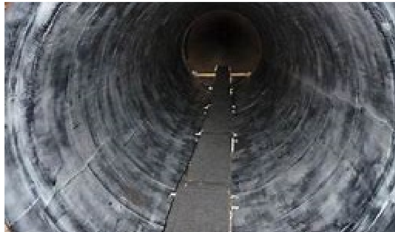
Longitudinal Crack observed at the invert of Pipe 8019 pipe
